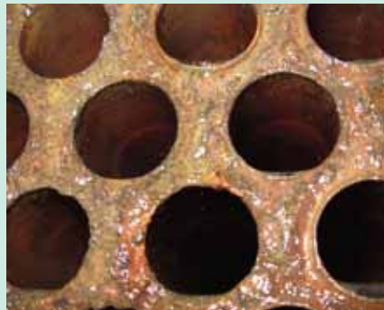
Photos • Left Hand View: 10-27-2005, algae before eH 2 O treatment and gone after treatment. Above: 11-7-2008, close up showing clean tubes without any brushing. The normal deposits from the tower on the tube sheet wipe off, showing nothing was touched on condenser. Above Right: Closing condenser right after inspection.
