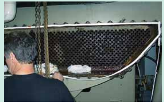
Photos • Left Hand View: 10-27-2005, algae before eH 2 O treatment and gone after treatment. Above: 11-7-2008, close up showing clean tubes without any brushing. The normal deposits from the tower on the tube sheet wipe off, showing nothing was touched on condenser. Above Right: Closing condenser right after inspection.
