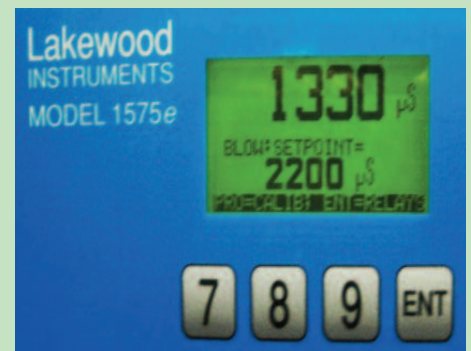
Above: 2200 set point running at 1330 is zero H 2 O discharge.
