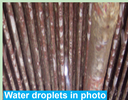
Above: Coil cleaning after just one month of Hybrid treatment.
